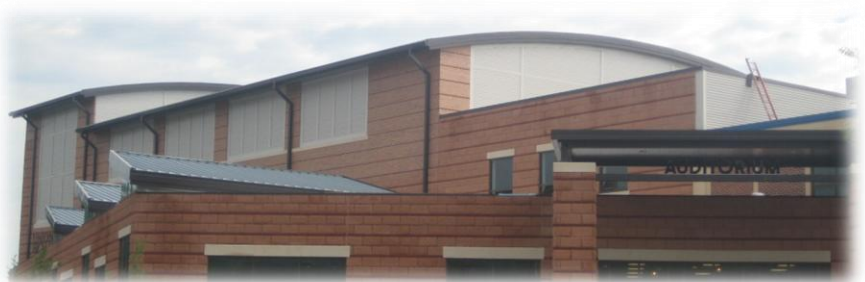
Figure 3: Barreled Auditorium Roof
