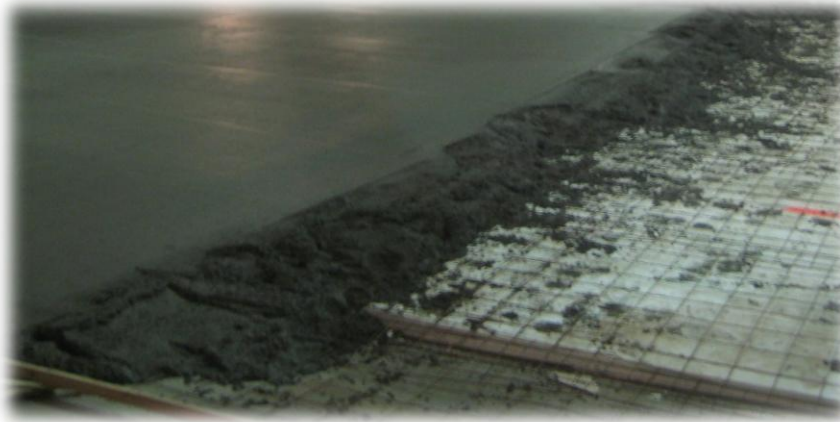
Figure 4: New Floor: Concrete over Geofoam Blocks
